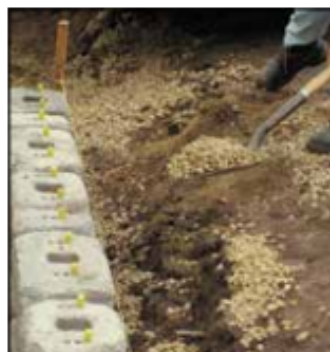
4. Install Fill & Compaction
